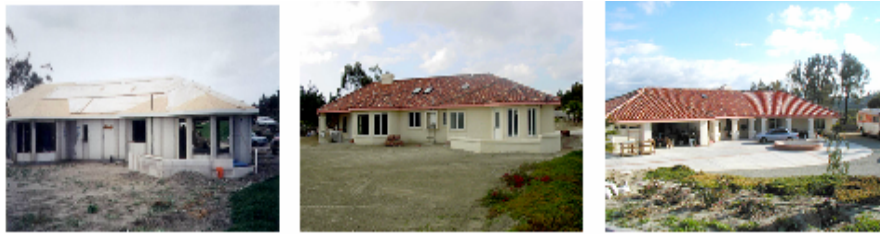
Figure 7: Complete roof load trusses setting on 3-D Panels [6].
