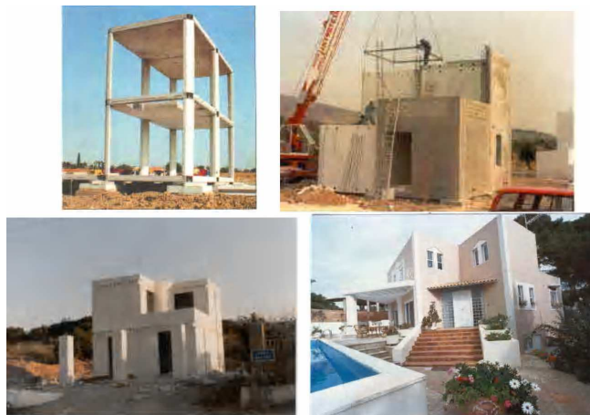
Figure 9: The first approach for a IBS panels, the prefabrication of entire cubes with lightconcrete and the assemblage of cubes into luxurious home [7].
