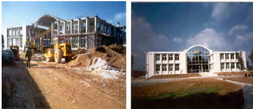
Figure 10: The 5000 m 2 administration office for (Athens International Airport) in Spata was planned and constructed in a period of 3 months [7].
