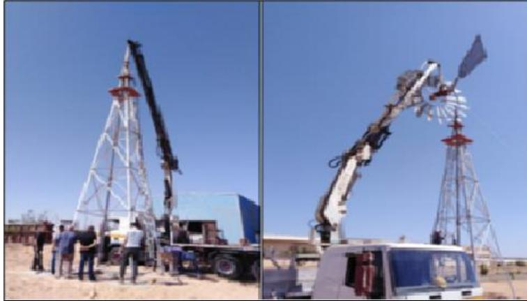
**Figure 18. Rotor and tower installation.**
