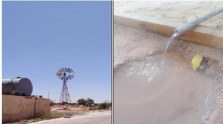
**Figure 19. Water is extracted from the Well by the windmill system.**
